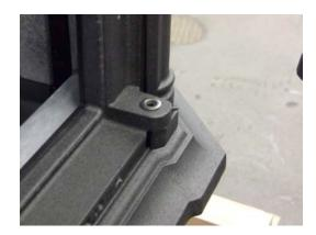
3. Lay the door, stone side down on a flat surface. Remove the four allen head bolts with a 5/32" hex key.
